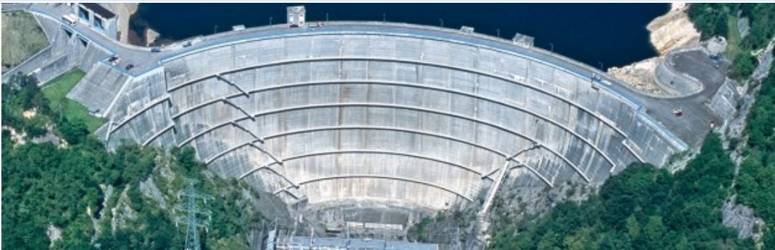
Multi-purpose Yagisawa Dam upstream in Tone River started construction in 1959 completed in 1967 131m high concrete arch dam, Japan Water Agency
