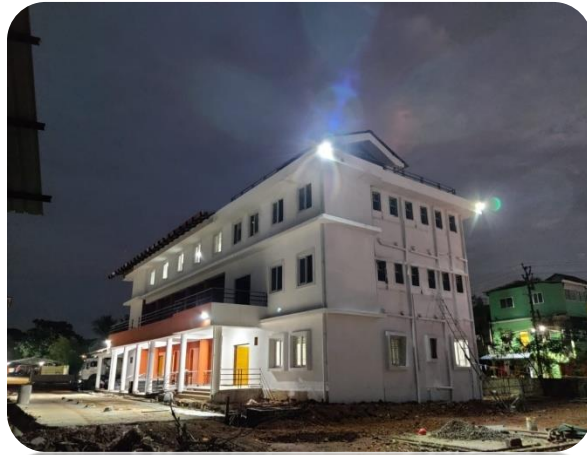
Multi Purpose Cyclone Shelters (MPCS)
