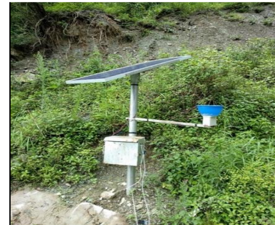
Installed Low Cost Sensors
