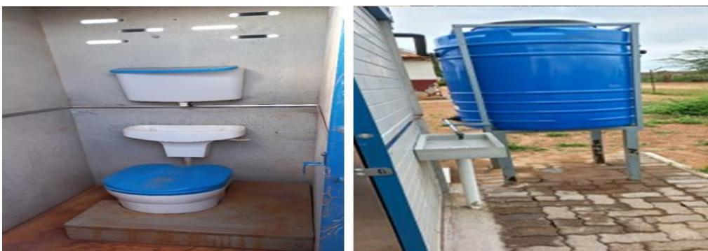
Figure 5: Newly constructed ablutions as part of the SAFE Schools Programme, LP
