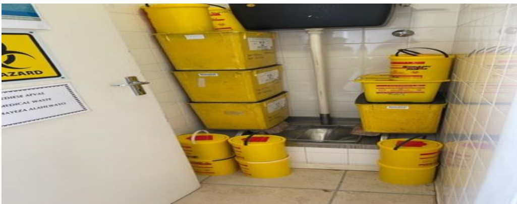
Figure 4: Inadequate medical waste storage at Heidelberg Clinic, WC
