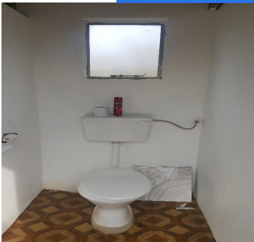
INTERIOR :ABLUTION FACILITIES FUNDED BY COGTA
