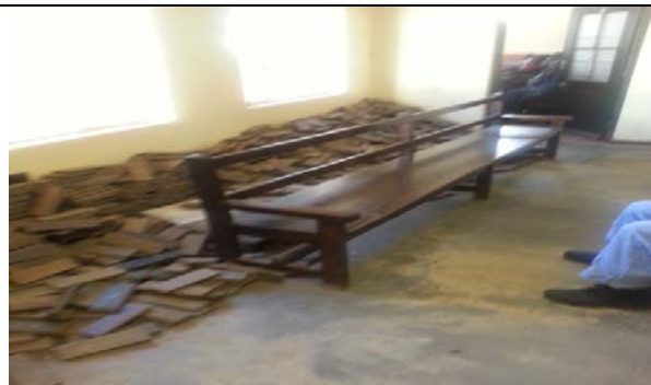
Figure : Pile of floor tiles in Mqanduli Magistrate Court, 2015
