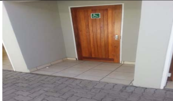
Figure : Ablutions for persons with disabilities at Barkley East DLTC, 2015
