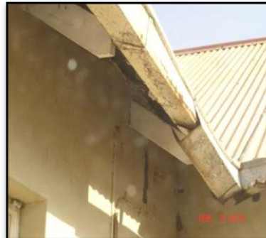
Mafani Clinic (FS): Broken fencing at (Left), and Viljoenskroon MCCC (FS): Broken gutters at (Right)
