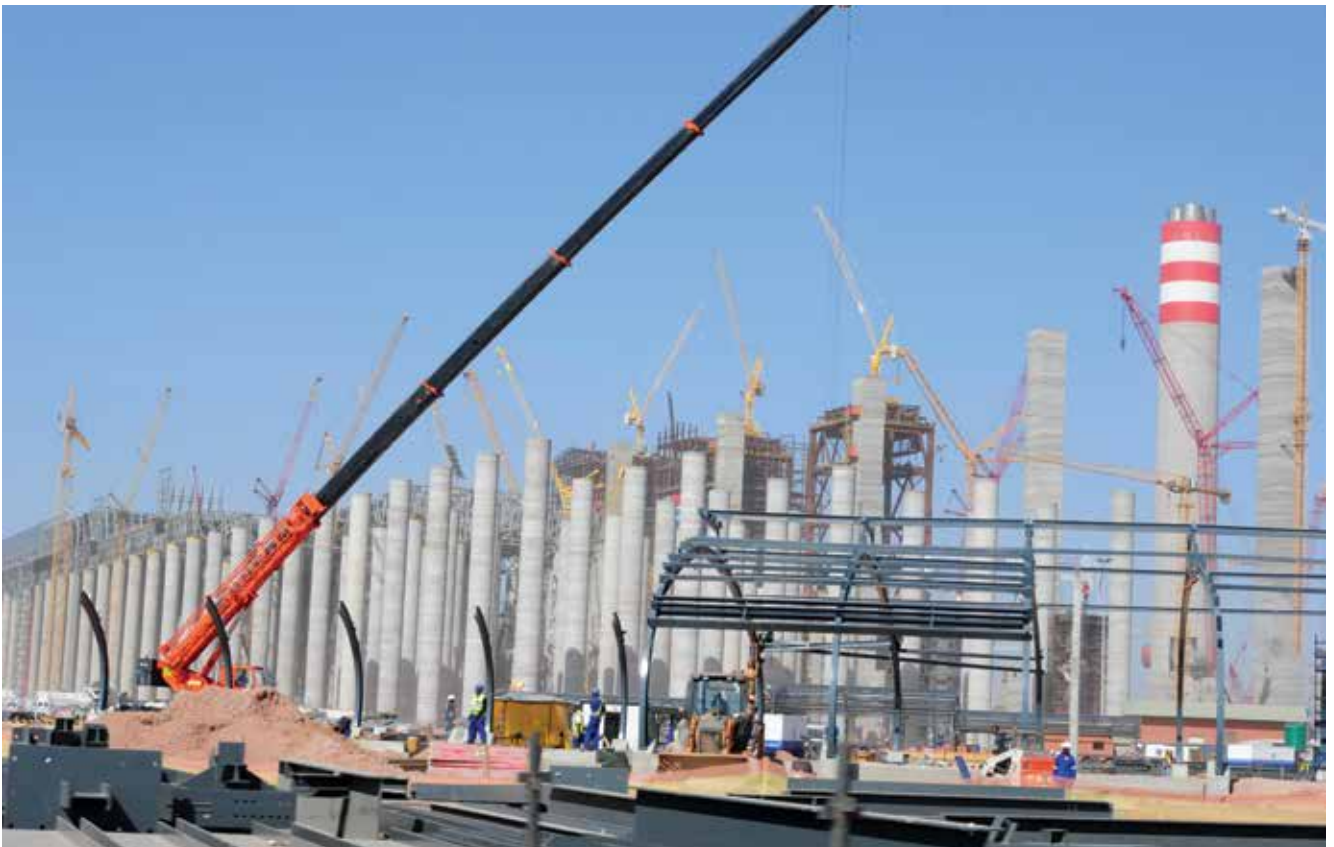
Construction of Medupi power station
